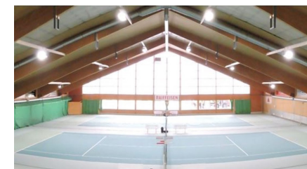
Tennishalle fitnxx Balsthal
